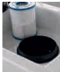
4. Remove the old filter and insert the replacement; repeat the previous steps
